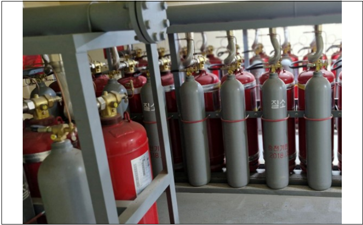
12 Gaseous Flooding System Bottles
