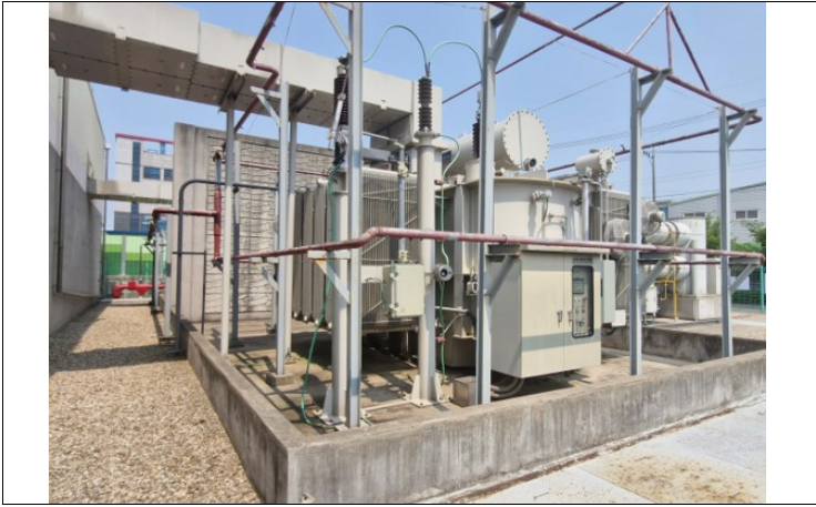
09 Fire Detection and Protection for Main TR
